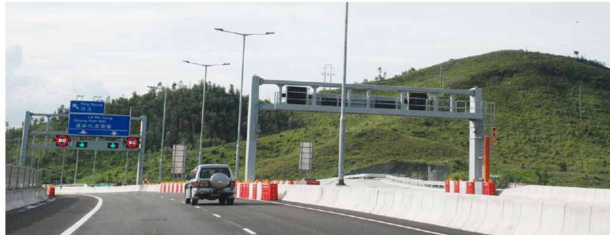
Hydroseeding on Slope (OM7) Tree Planting on Landscape Slope (OM3 & 7)
