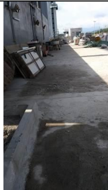
The chemical containers were removed.
