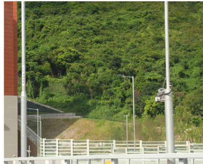
Buffer Trees Planting with Amenity Shrubs Planting (OM3 & 4) Tree Planting on Landscape Slope (OM3 & 7) Berm Planter on Slope (OM2 & 7)
