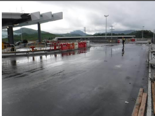
The cement mixing plant were removed.
