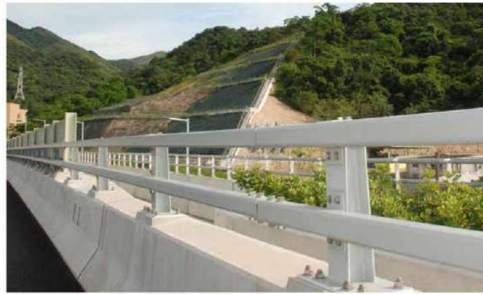
Hydroseeding on Slope (OM7)
