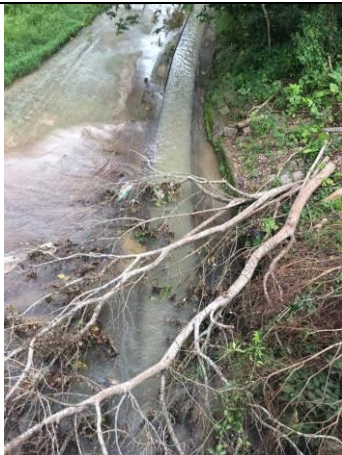
Photo 3 On 1 August 2019, turbid water was observed at WM3x.
