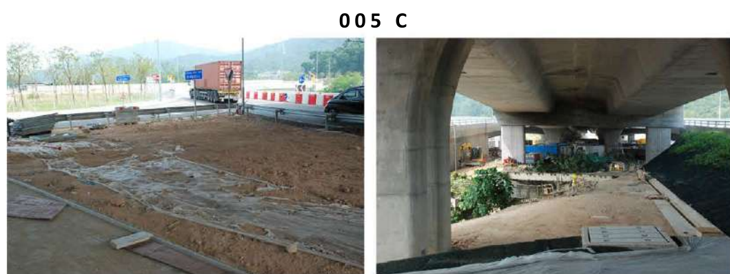
005 C Amenity Improvement Planting under Viaduct (Hydroseeding and Climbers) (OM6)
