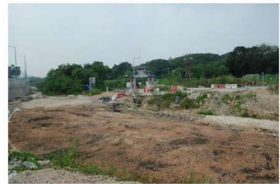
Buffer Trees Planting with Amenity Shrubs Planting (OM3 & 4) Amenity Roadside Trees Planting (OM3 & OM10)
