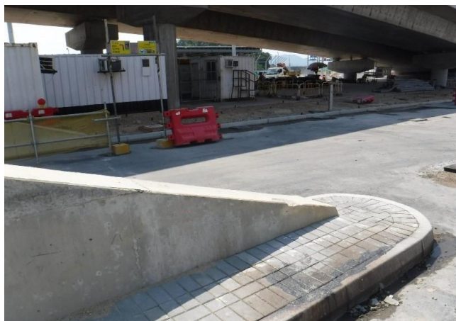
Chemical container was removed.
