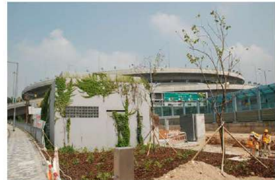
001 D Existing Pumping Station
