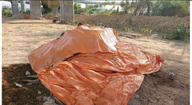
The stockpile was covered with tarpaulin sheets properly.
