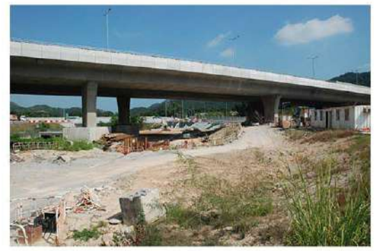
Buffer Trees Planting with Amenity Shrubs Planting (OM3 & 4) Tree Planting on Landscape Slope (OM3 & 7)
