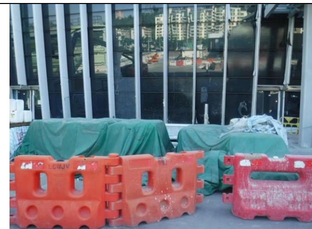
The cement bags were covered with tarpaulin sheet.
