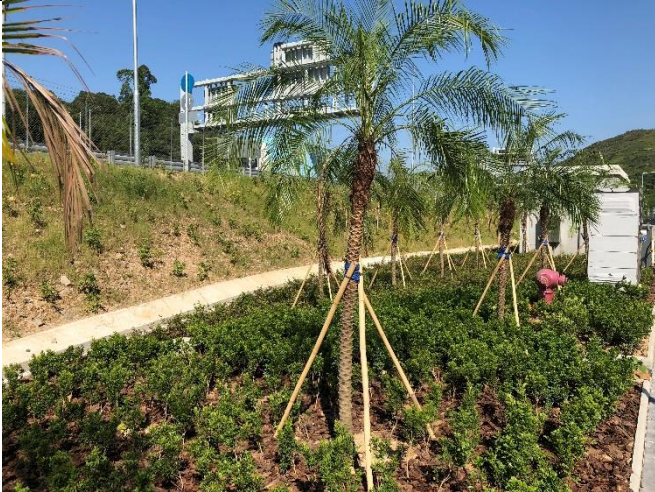
Hydroseeding was applied on the exposed wore area.
