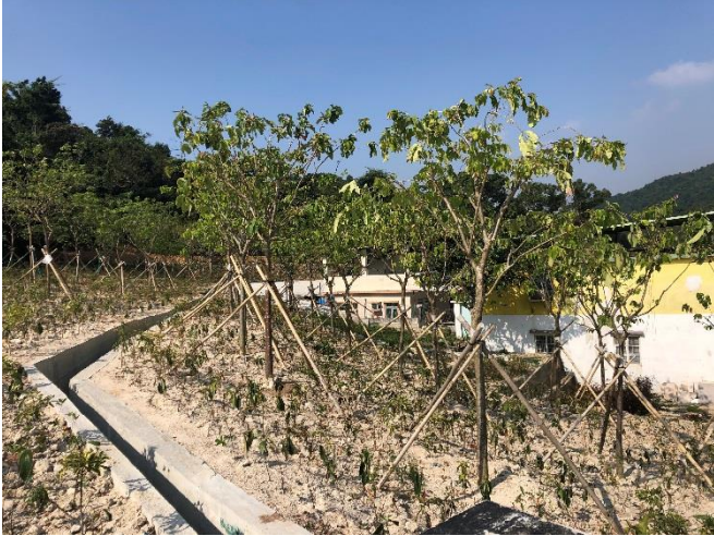
Hydroseeding was applied on the exposed work area.
