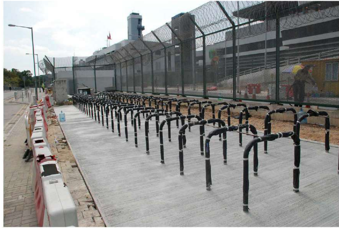
Cycle Parking Facilities
