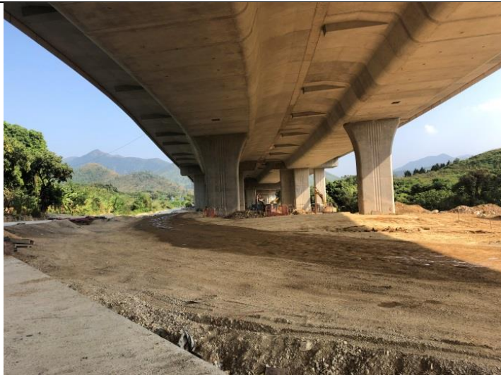
Photo 1 Overview of Wetland Compensation Area (WCA)
