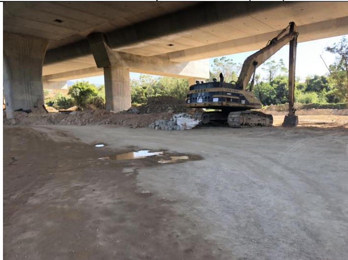
Photo 3 Excavation of the proposed pond was observed at WCA.
