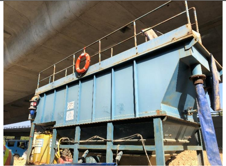
Photo 2 Wastewater treatment facility was implemented at WCA.
