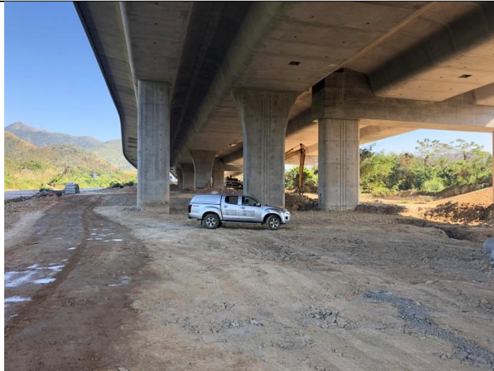
Photo 1 Overview of Wetland Compensation Area (WCA)
