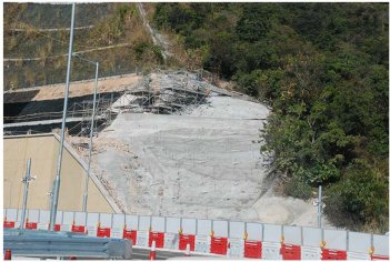
Berm Planter on Slope (OM2 & 7)
