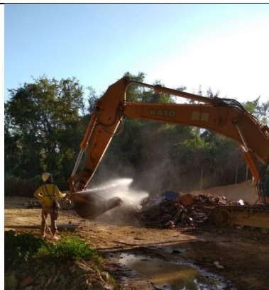
Water spraying was provided onsite.
