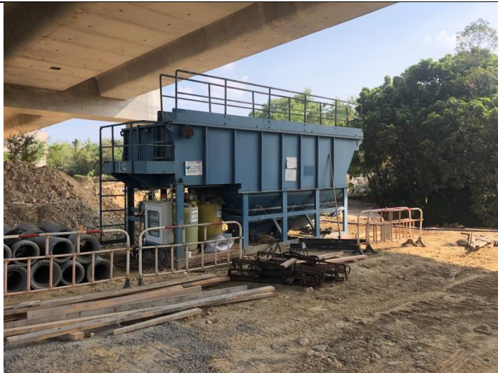
Photo 3 Wastewater treatment facility was assembled at WCA.
