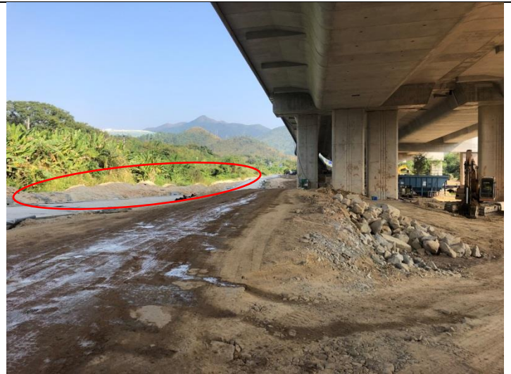
Photo 2 Preparation work and exportation of soil stockpiled in WCA were observed.
