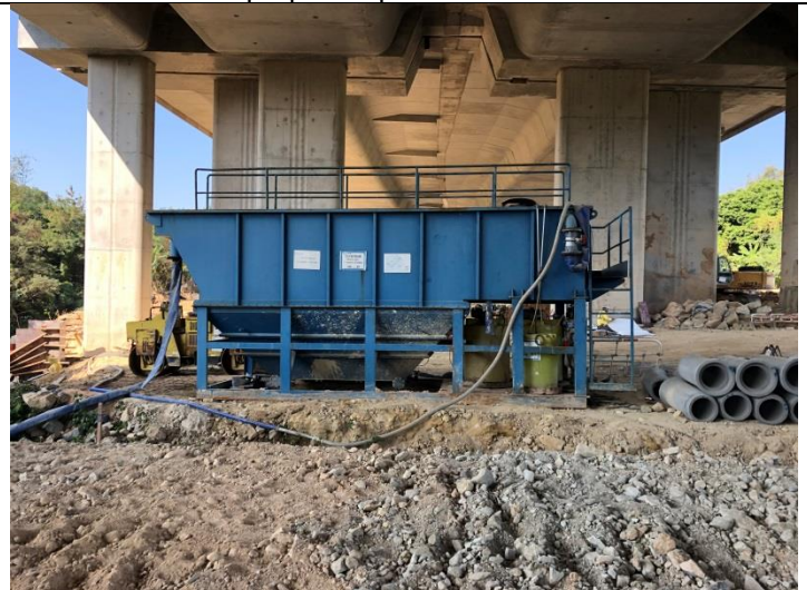
Photo 4 Wastewater treatment facility was implemented at WCA.
