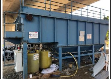
Photo 3 Wastewater treatment facility was implemented at WCA.
