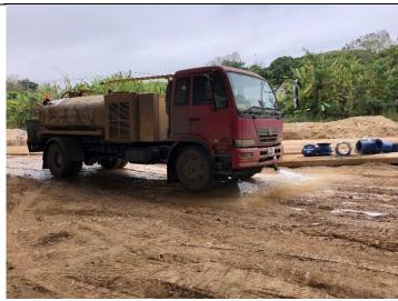
Photo 5 Water spraying was implemented on site to reduce dust dispersion.
