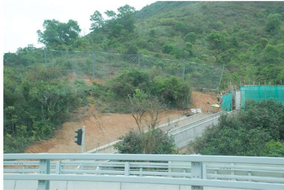
Woodland Mix Planting on Slope (OM3 & 7) Flexible Barrier
