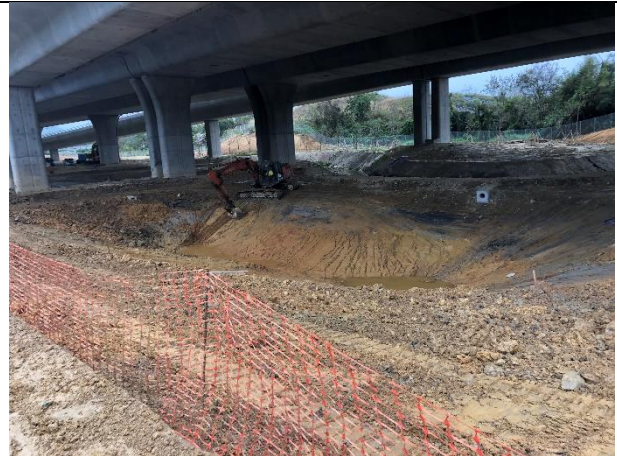
Photo 2 Excavation of soil at pond D was observed at WCA.
