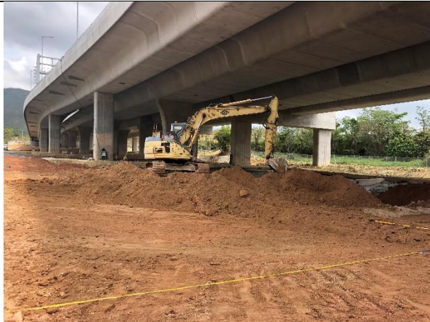
Photo 1 Soil laying at the proposed pond at WCA.
