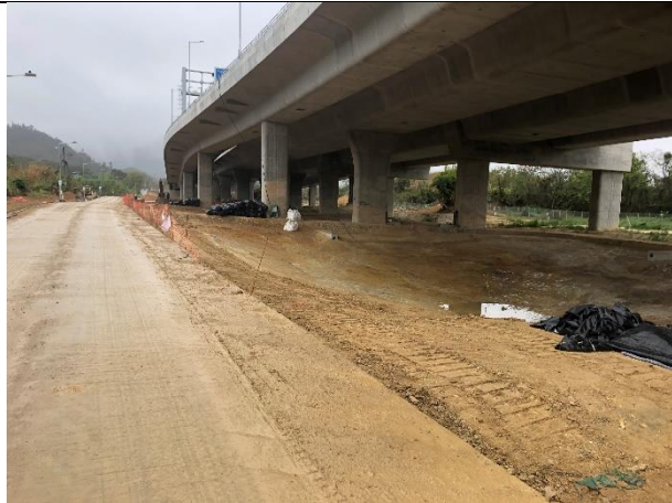
Photo 1 Overview of Wetland Compensation Area (WCA)
