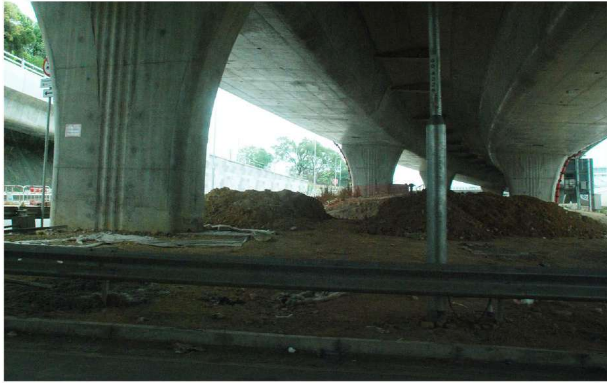
Amenity Improvement Planting under Viaduct (Hydroseeding and Climbers) (OM6)
