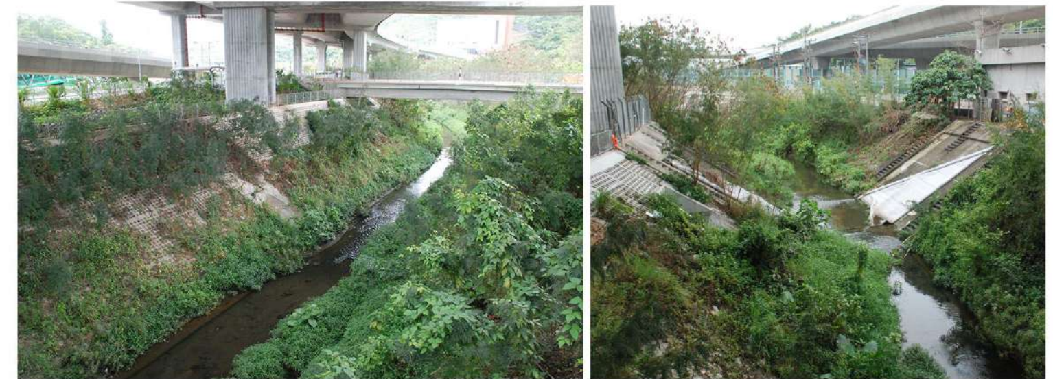
Existing River Bank/ Channel Bank to be Retained (OM11)
