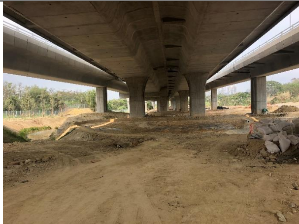
Photo 1 Overview of Wetland Compensation Area (WCA)
