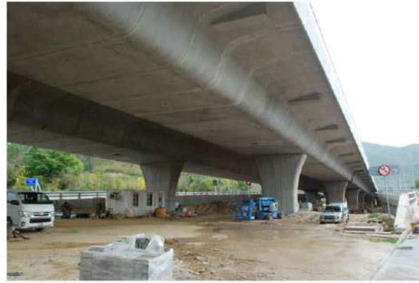
Amenity Improvement Planting under Viaduct (Hydroseeding and Climbers) (OM6)
