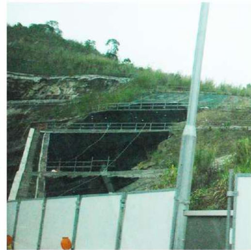
Berm Planters on Slope (OM2 & 7) Shrubs and/or Groundcover Planting on Slope (OM7)
