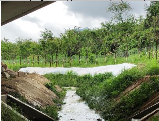
Photo 3 Hydroseeding was applied on the exposed work area.
