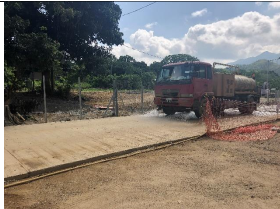
Photo 4 Water spraying was provided on the haul road at WCA.
