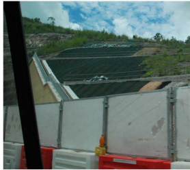
Berm Planters on Slope (OM2 & 7) Shrubs and/or Groundcover Planting on Slope (OM7)
