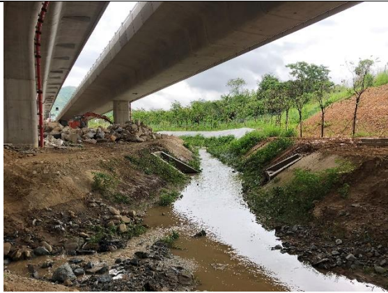
Hydroseeding was applied on the exposed slope.
