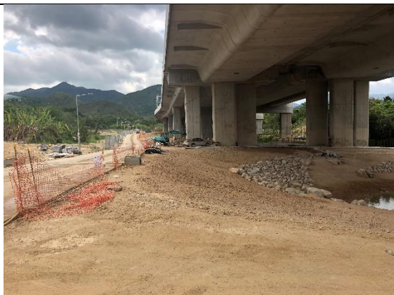
Photo 3 Overview of wetland compensation area(WCA).
