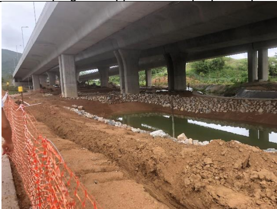
Photo 3 Overview of wetland compensation area (WCA).
