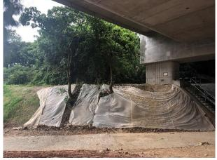
Hydroseeding was applied on the exposed slope.
