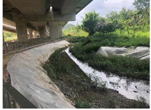
**Photo 3** Hydroseeding was applied on the exposed slope at WCA.
