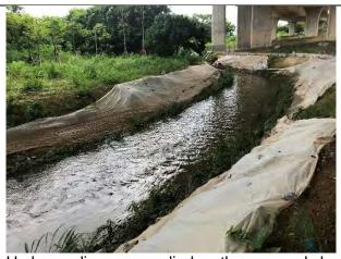
Hydroseeding was applied on the exposed slope.
