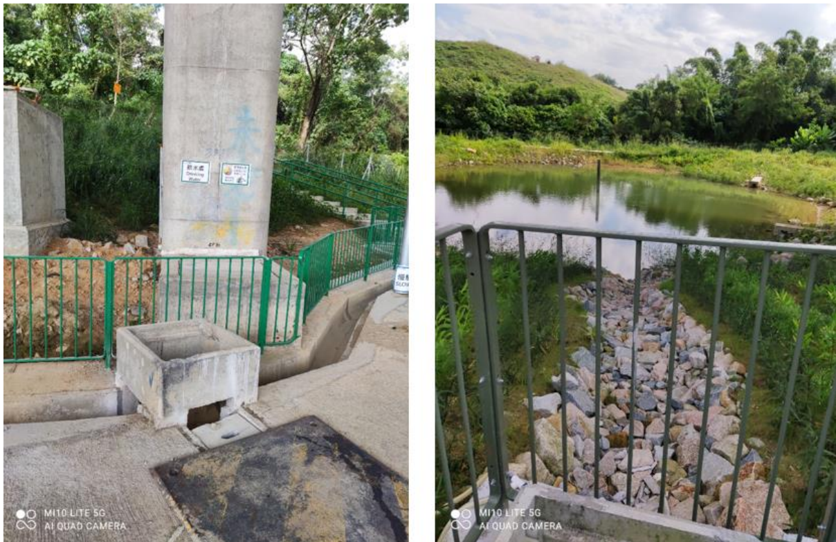
Figure 2-14 The 300mm U-Channel, Catchpit, and Rock Channel
