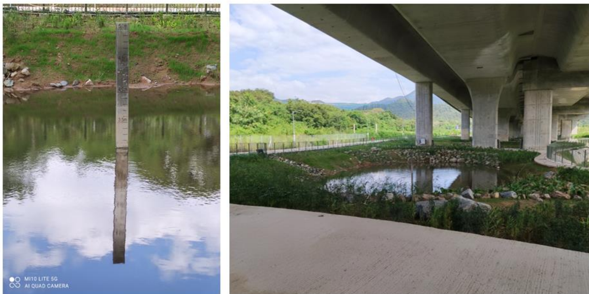
Figure 2-8 The Site Visit Dated 16 th Oct 2020 (Typical Dry Season)
