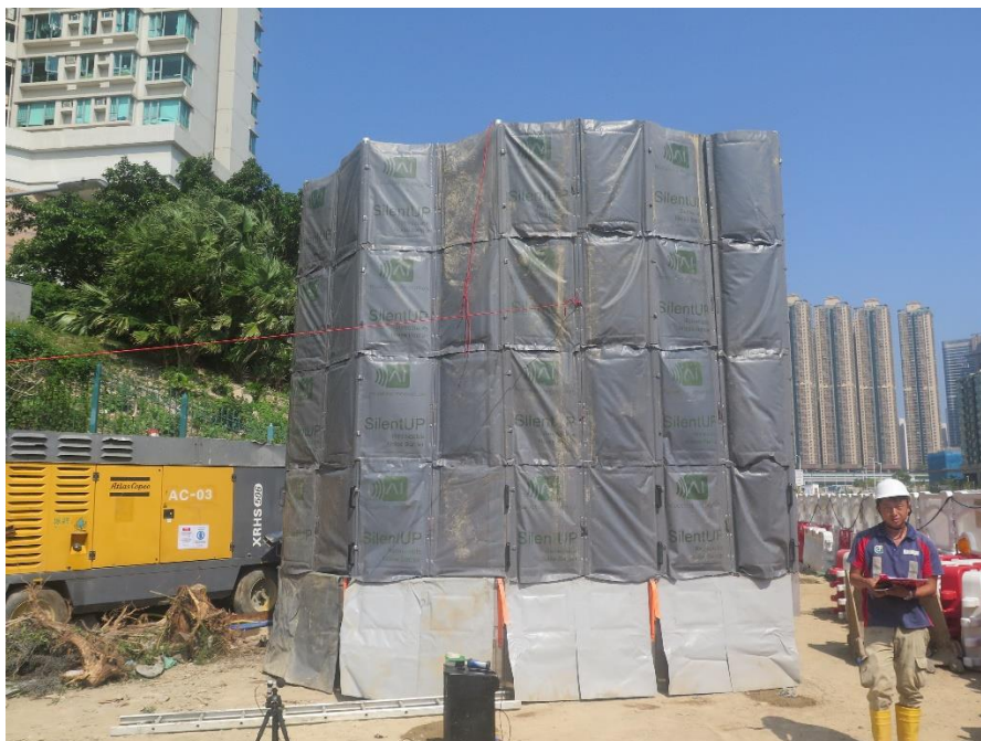
Photo 1. Noise Barrier (front view)
