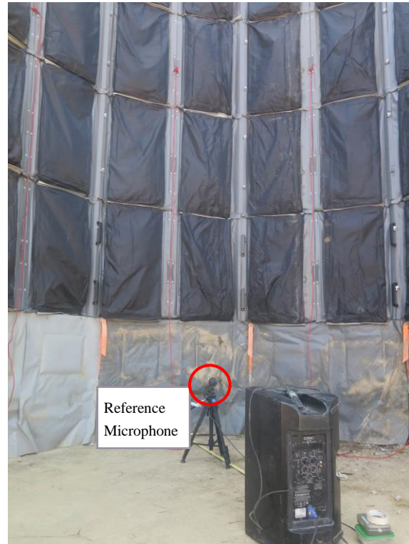
Photo A2. Loudspeaker, Reference Microphone and Enclosure for with Noise Barrier Scenario
