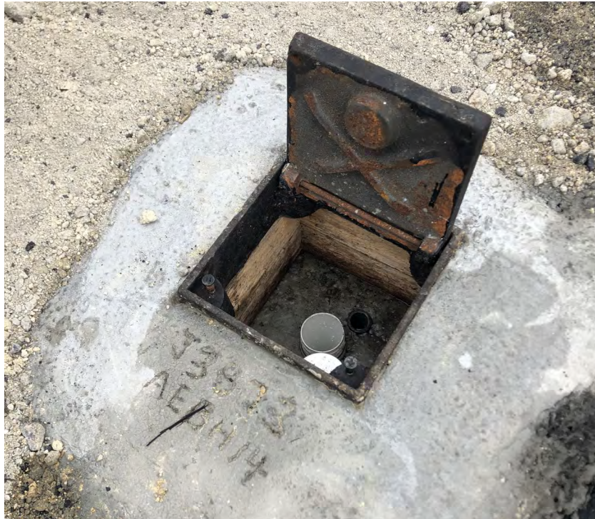
Photo 7: Groundwater well installation
