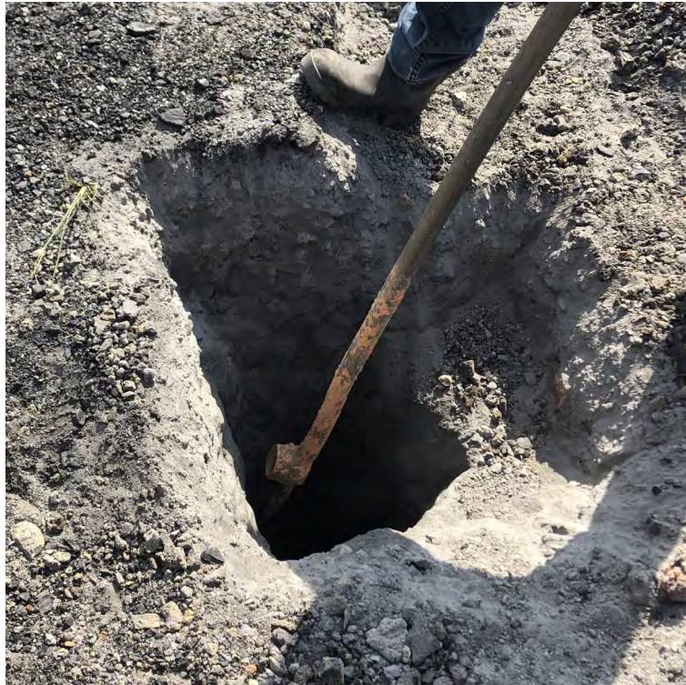
Photo 1: Inspection Pit at AEBH20
