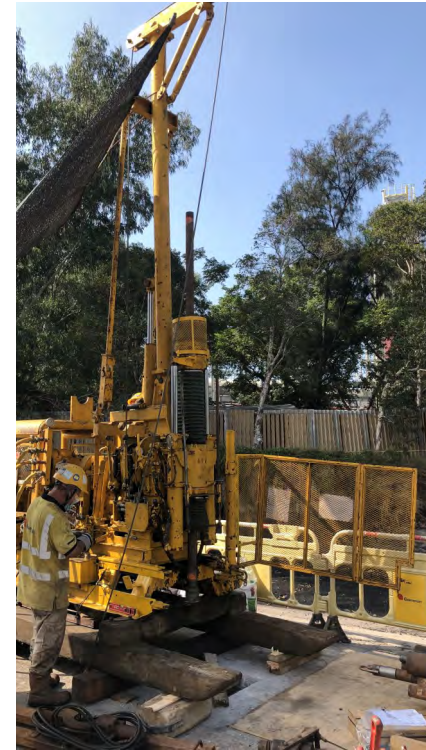
Photo 4: Borehole drilling at AEBH21
