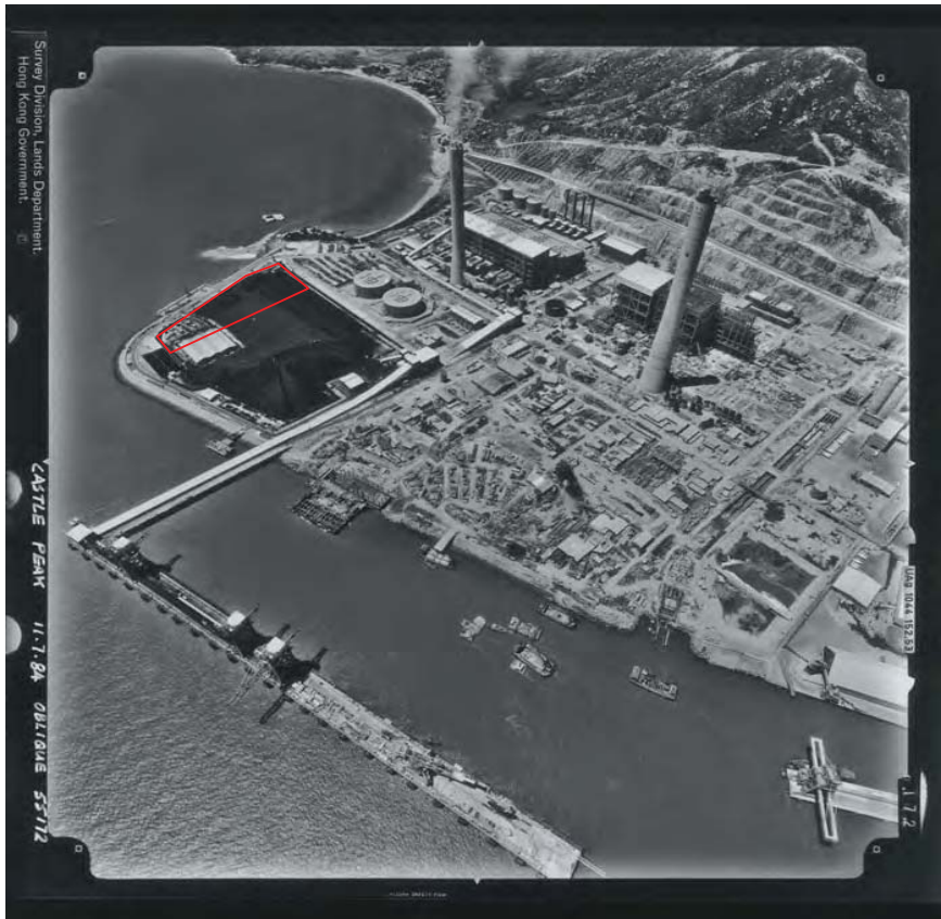
Year 1984 (ref: CS17522): Part of the works area was constructed with three consecutive single - storey buildings which resembled warehouses / workshops. The West Coal Stockyard was established.
