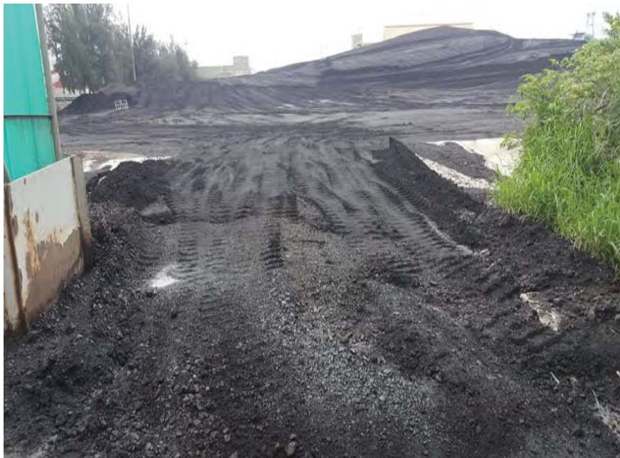
Photo 1: Entrance of west coal stockyard. The area is covered with coal pile.
