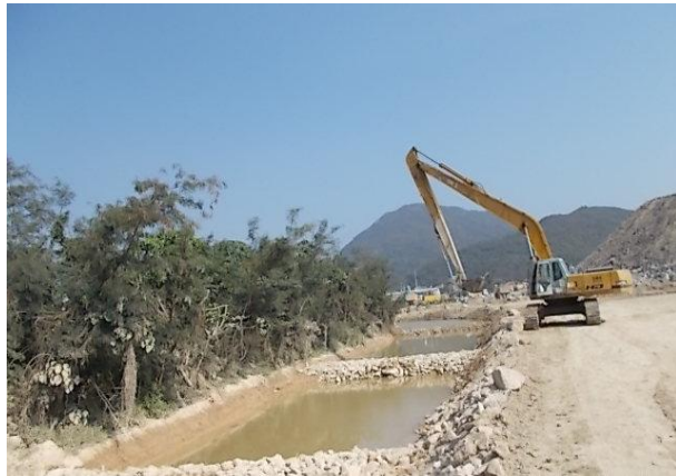
Drainage system were adequate and well maintained to prevent flooding and overflow.
