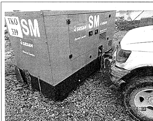
Photo 190527_001 (Near Asphalt Deposition Platform) (Improved)
