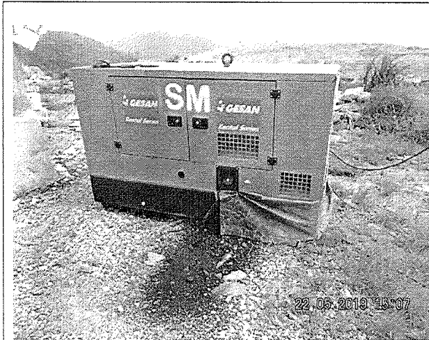
Photo 190522_001 (Near Asphalt Deposition Platform)
