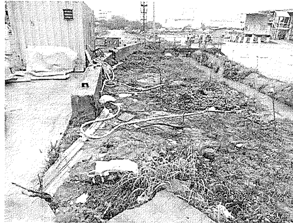
Photo 200318_002 (Near Dewatering pound)
