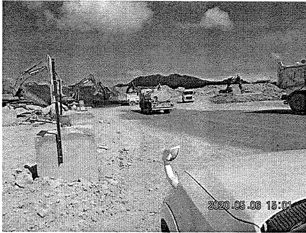
Photo 200506_001 (Near 3RS soil platform)(Improved)
