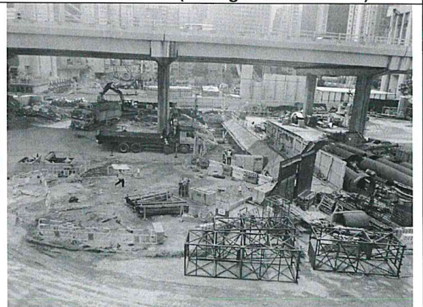
Photo 4 - Private Project Site to Harbour Grand HK Hotel (Wan Wah Mansion behind the Hotel)
