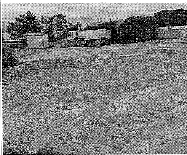
Photo 220131_001 (Near Workshop) (Improved)
