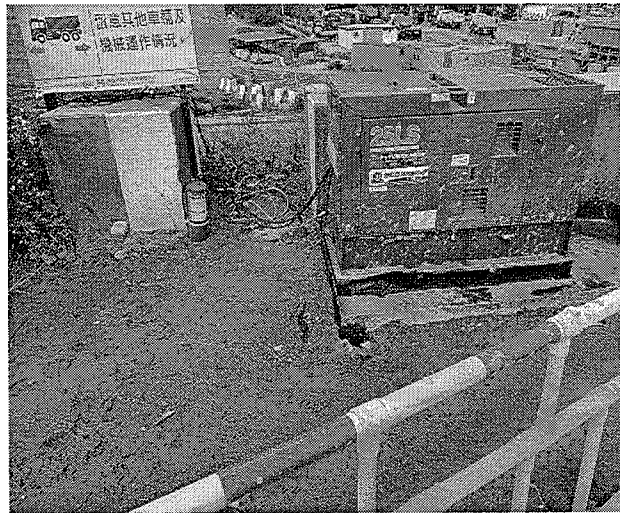
Photo 220119_001 (Near Fixed Rigid Platform) (Improved)
