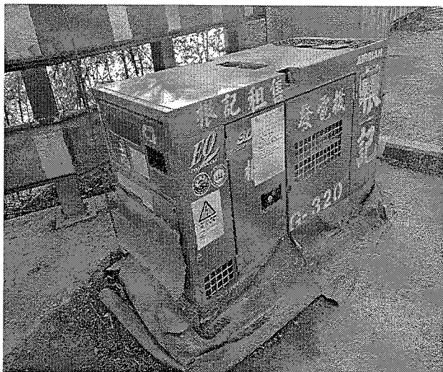
Photo 211118_001 (Near No.1 tipping hall)
