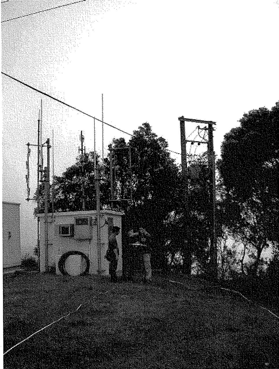
Picture 2: General View of the Existing Radio Equipment Room
