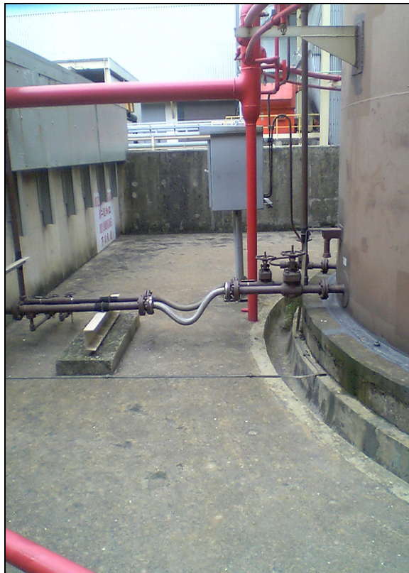
Photo A2 The Pipe Work within the Bunded Area shows no Visible Staining.
