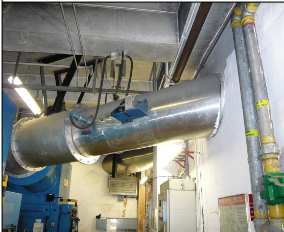
Horizontal flue in the incinerator room
