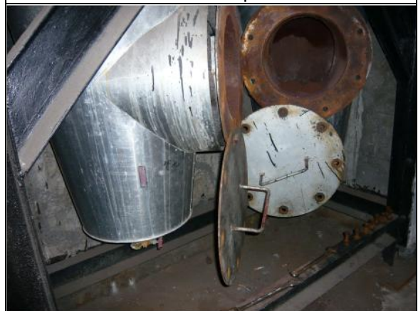
Ash collectors at the bottom of the chimney
