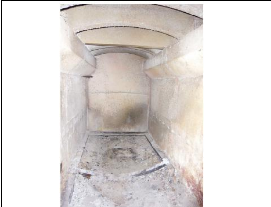
Residual ash in incinerator 1
