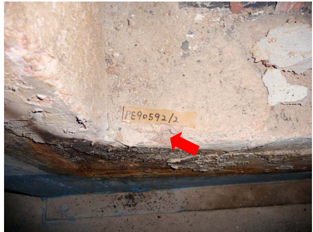
Photo 2. Insulation Brick (PE90592/2) sampled at Incinerator 2, Incinerator Room, B/F was confirmed as Non-ACM.
