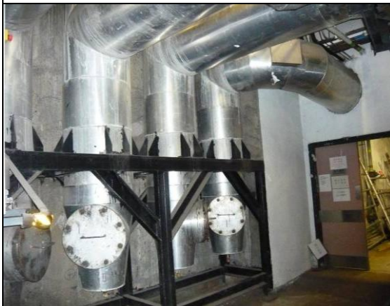
Horizontal flue joining the vertical chimney section (2 flue for incinerator at the far right, 2 flue nearest for the boiler)
