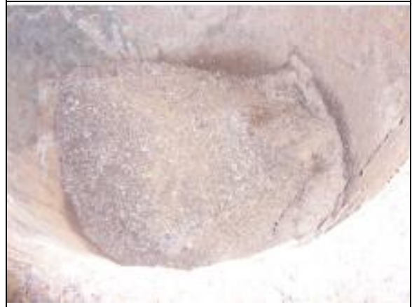
Residual ash in the ash collector (bottom of chimney)
