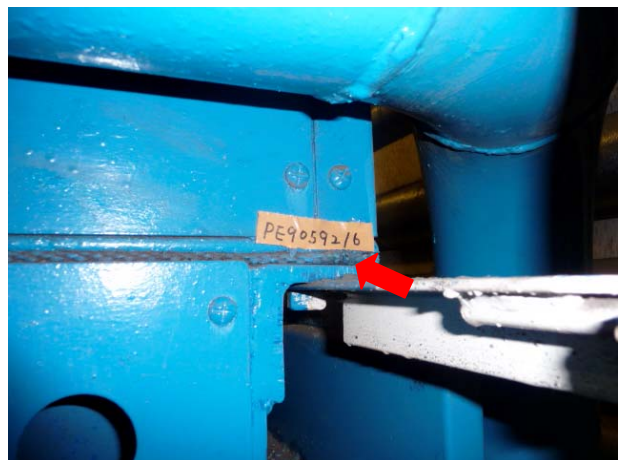
Photo 6. Incinerator Insulation (PE90592/6) sampled at Incinerator 2 was confirmed as Non-ACM.
