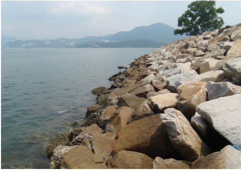
Artificial sloping boulder-mounted seawall at Site R3
