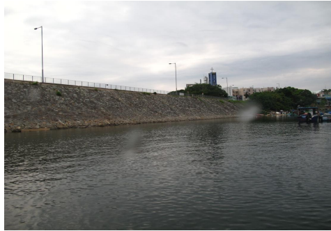
The artificial sloping at Site C2
