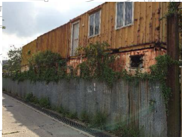
PHOTO 4: OUTSIDE SUSPECTED CARPARK / WORKSHOP (DATE TAKEN: 1 APRIL 2015)
