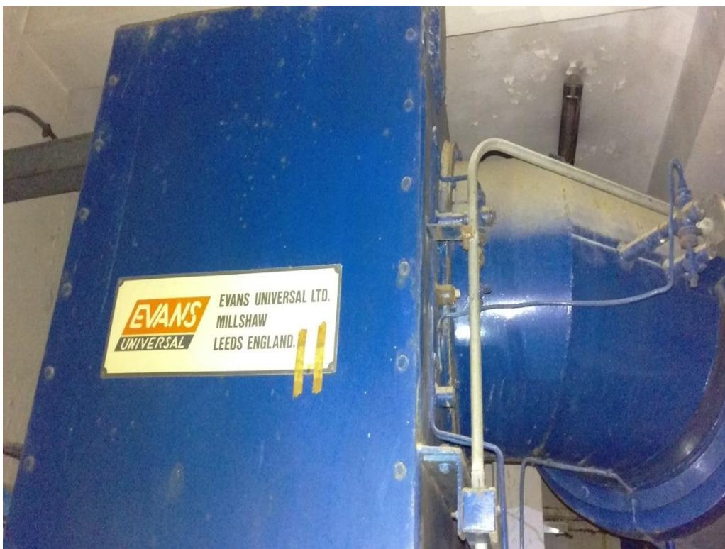
Plate 4 Upper part of the incinerator
