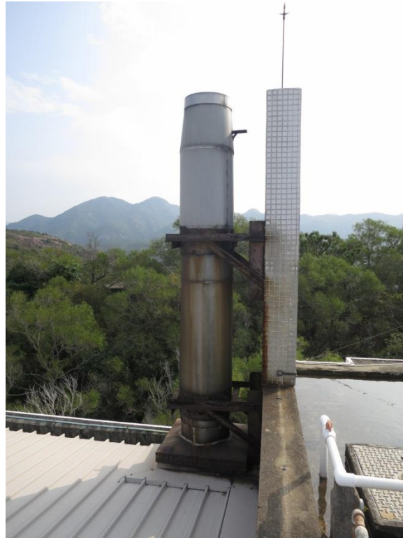
Plate 8 Chimney of the incinerator
