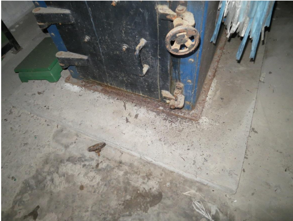
Plate 7 Ground slab for the incinerator
