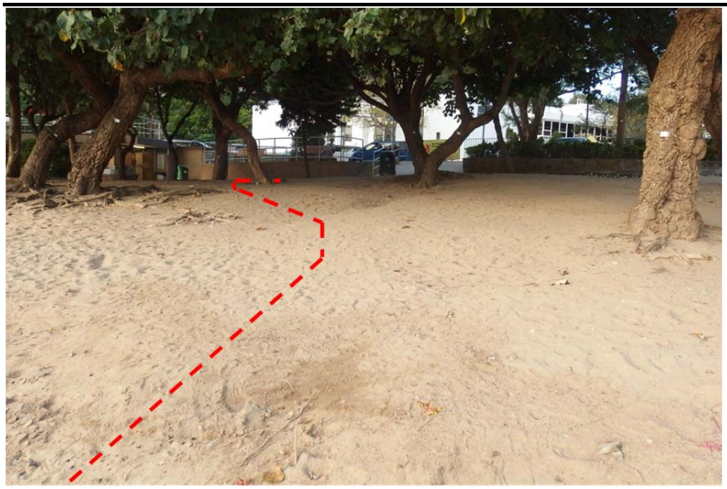
Figure 2.4 Proposed Route through Trees to BMH at DWB. Route to ensure Minimum Root Disturbance (Looking to Land)
