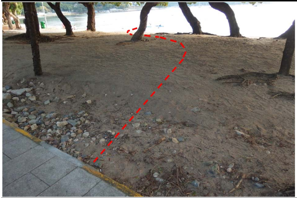
Figure 2.3 Key Area of Hand Dug Trench (Seaward) along Route to ensure Minimum Root Disturbance
