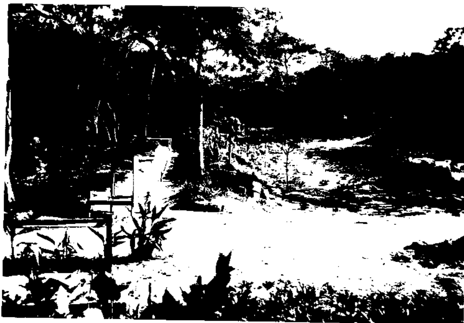
Photo 7 – U-channel along the site boundary together with the existing 2m-4m wide firebreak as left by the former army camp, effectively prevents the extension of fire hazards.
