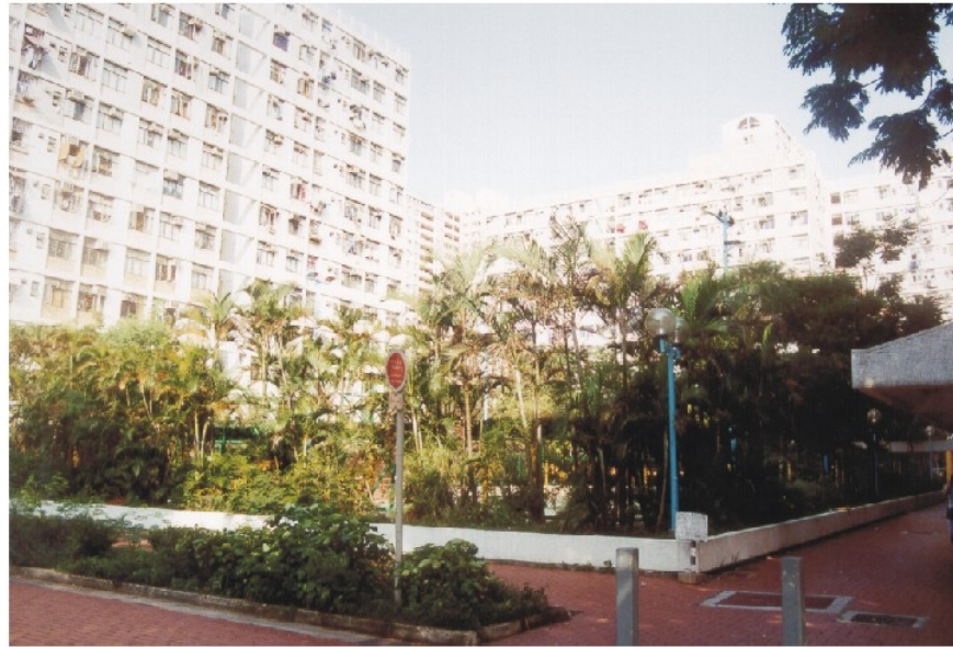
10. Typical View of Medium-rise Residential 2 (MR 2) showing open space at Tung Tau Estate which is generally hard but with mature planting
