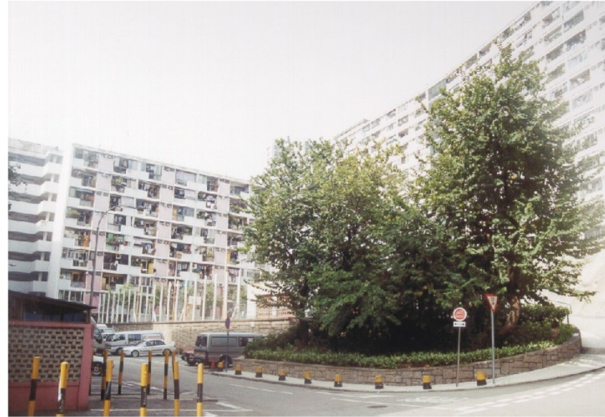
13. Typical View of Medium-rise Residential 5 (MR 5) showing Upper Ngau Tau Kok Estate. As with other older estate, the open space is primarily hard in character but has mature planting
