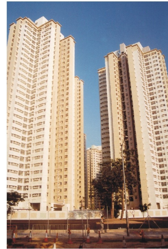
4. Typical View of High-Rise Residential 2 (HR 4) Showing the new residential developments with dense regimented layout
