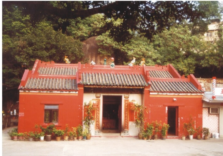
Typical View of the Temple in Medium-rise Residential 3 (MR 3) off Prince Edward Road East to the south-east of Choi Hung Interchange
