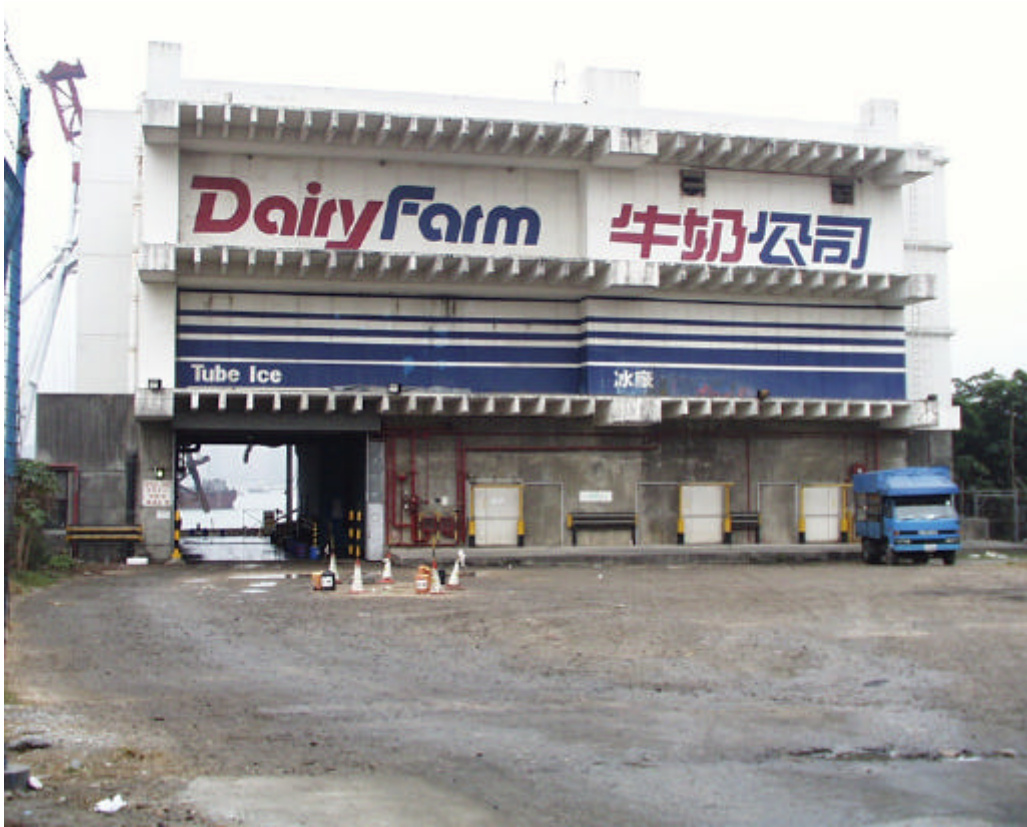
Photo 101 Existing Ice and Cold Storage Factory (17 Mar 99)
