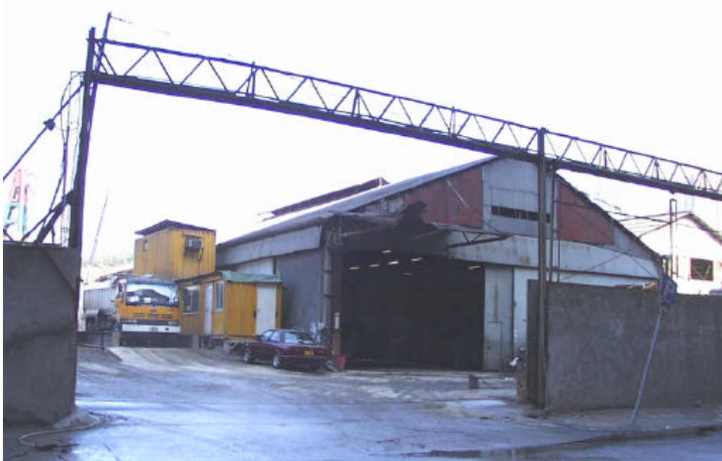
Photo 20 YTML 54 : Former ship repair workshop now occupied for construction material distribution and storage (5 Dec 98)
