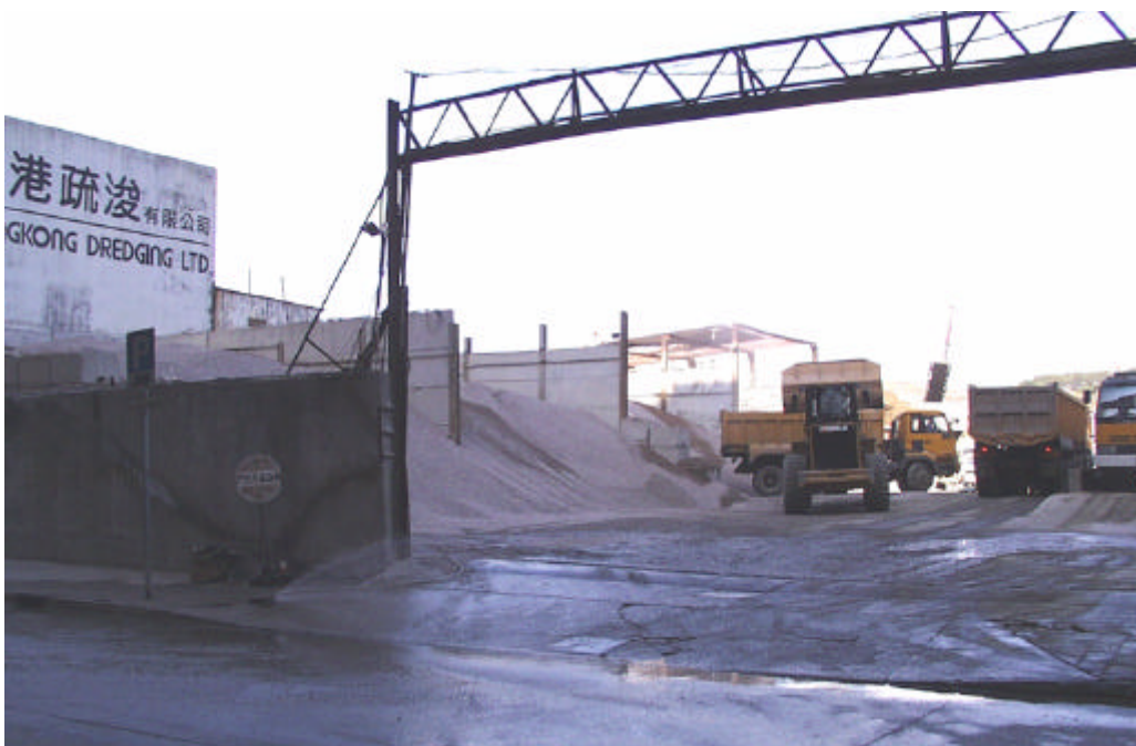
Photo 21 YTML 54 : Distribution and storage for construction material (5 Dec 98)
