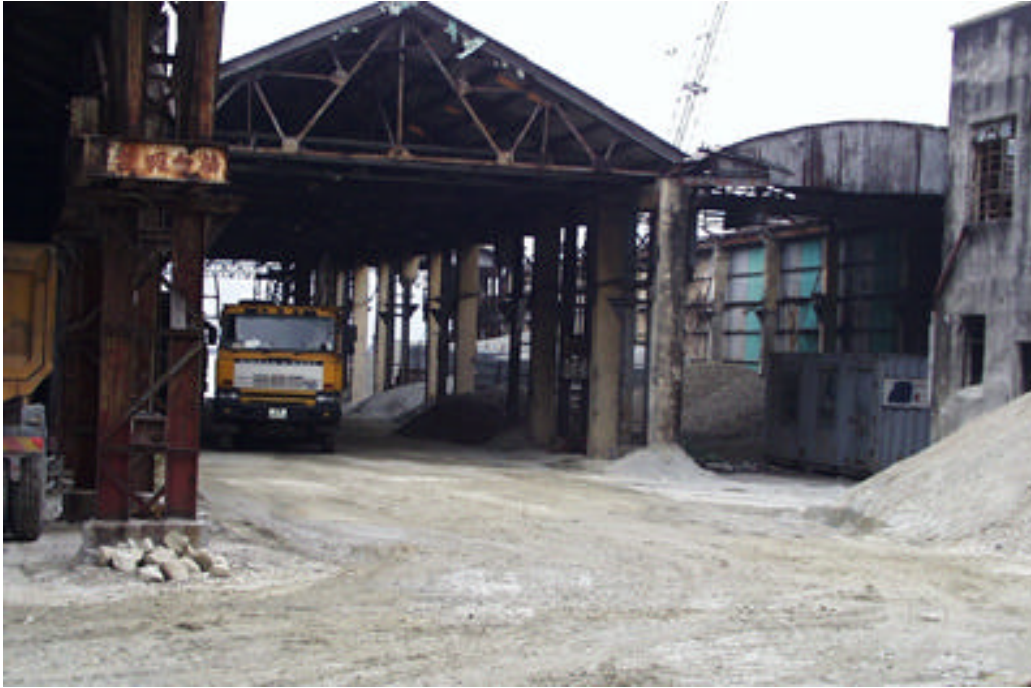
Photo 32 YTML 22RP, 23 to 24 : Storage for building materials (24 Dec 98)
