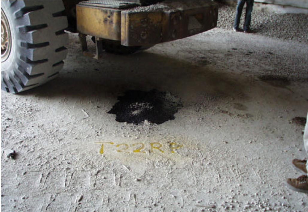
Photo 36 YTML 22RP, 23 to 24 : Oil spillage observed at the site (26 Jan 99)
