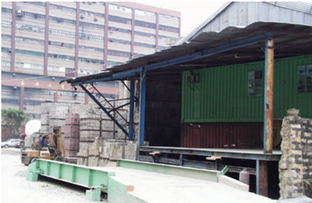
Photo 33 YTML 22RP, 23 to 24 : Storage for building materials (24 Dec 98)
