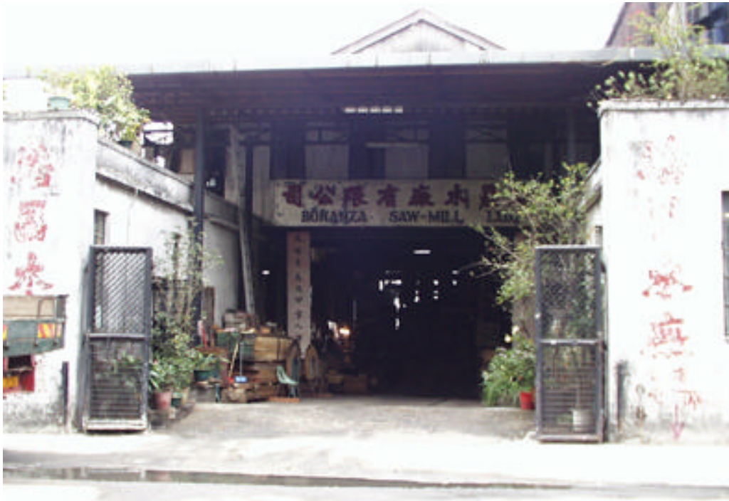
Photo 39 YTML 27 : Front view of the timber factory in operation (24 Dec 98)
