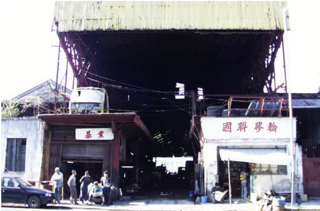
Photo 41 YTML 28 : Former sawmill used as car repair centre (5 Dec 98)
