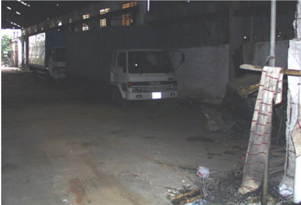
Photo 50 YTML 29 : Vacated timber factory (24 Dec 98)
