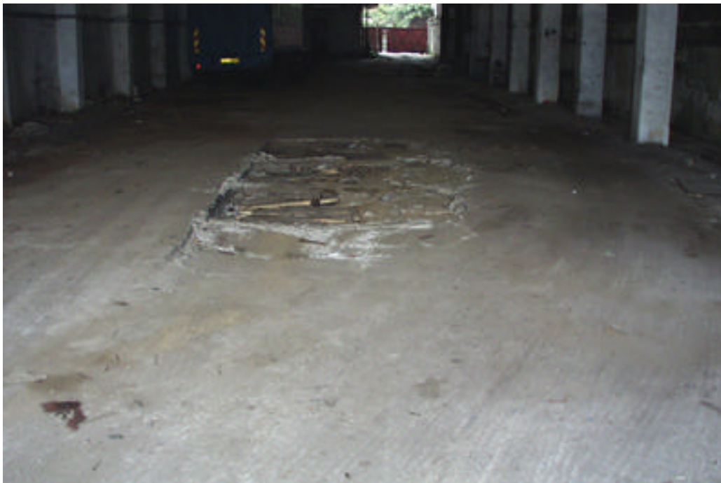
Photo 49 YTML 29 : Vacated timber factory (24 Dec 98)
