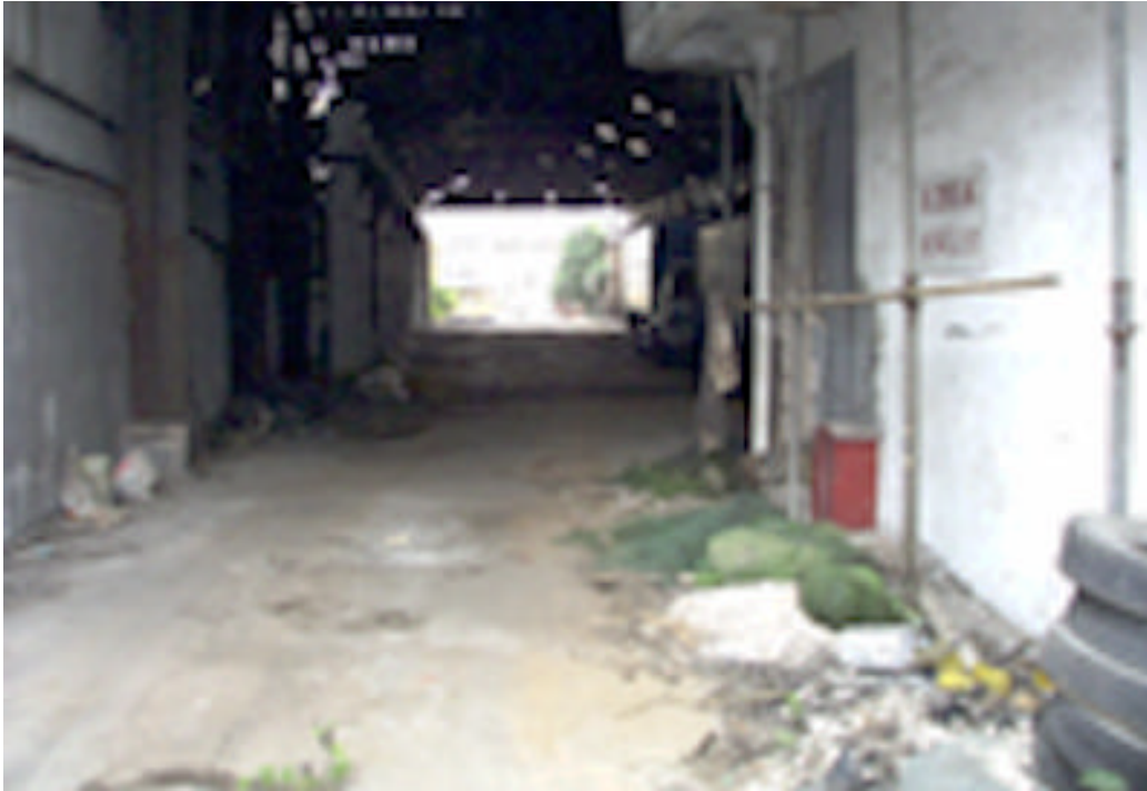
Photo 48 YTML 29 : Vacated timber factory (24 Dec 98)
