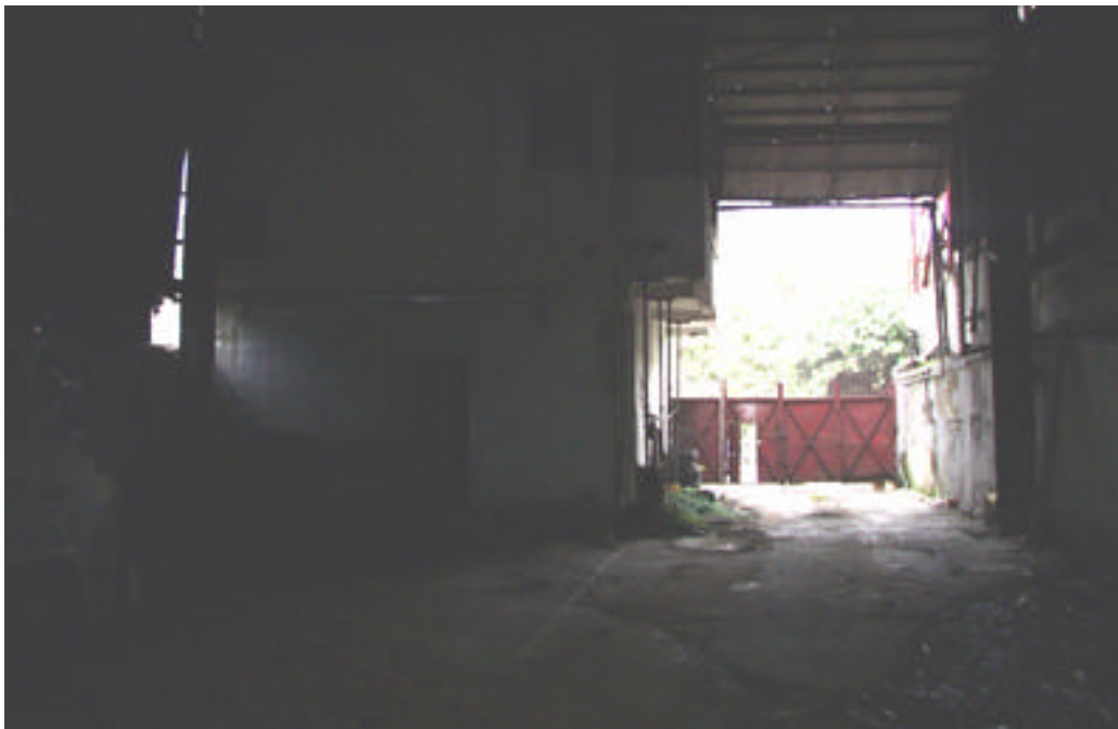
Photo 51 YTML 29 : Vacated timber factory (24 Dec 98)
