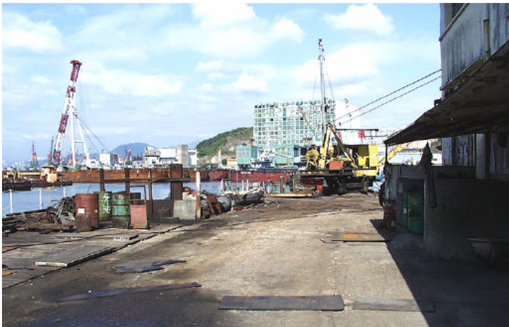
Photo 6 YTML 6-11 : Ship repair workshop in operation (5 Dec 98)
