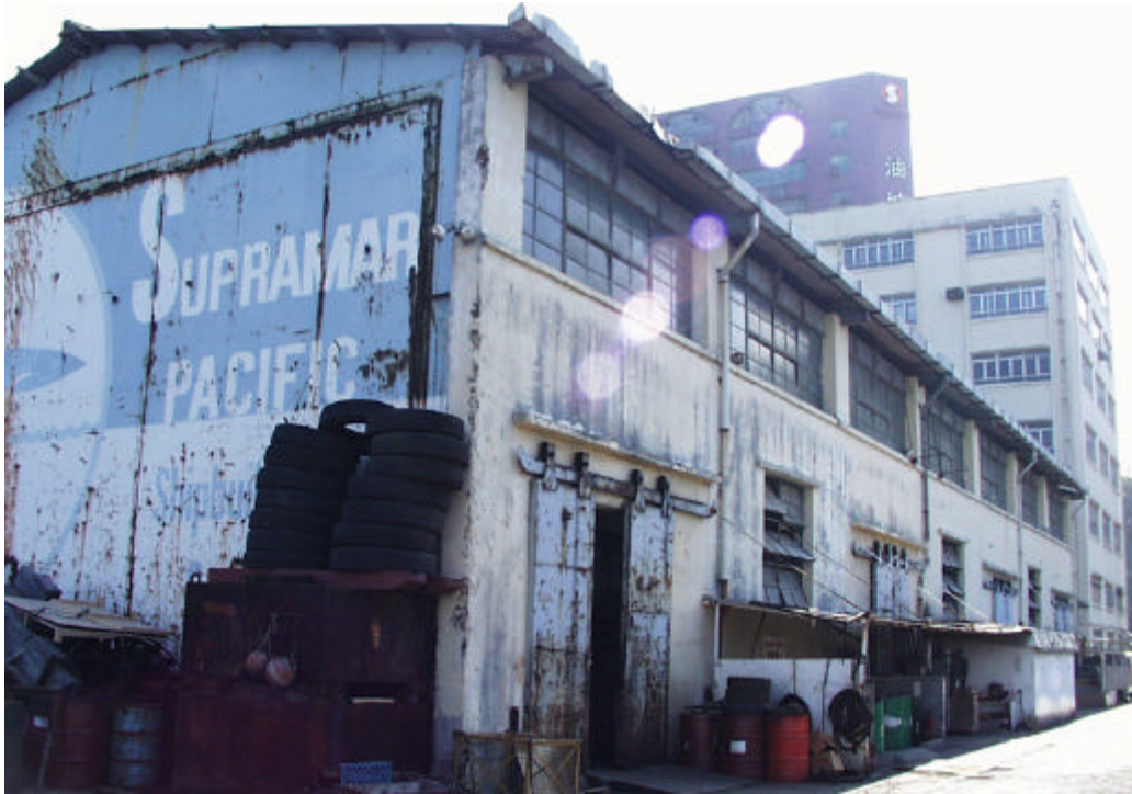
Photo 5 YTML 6-11 : Ship repair workshop in operation (5 Dec 98)
