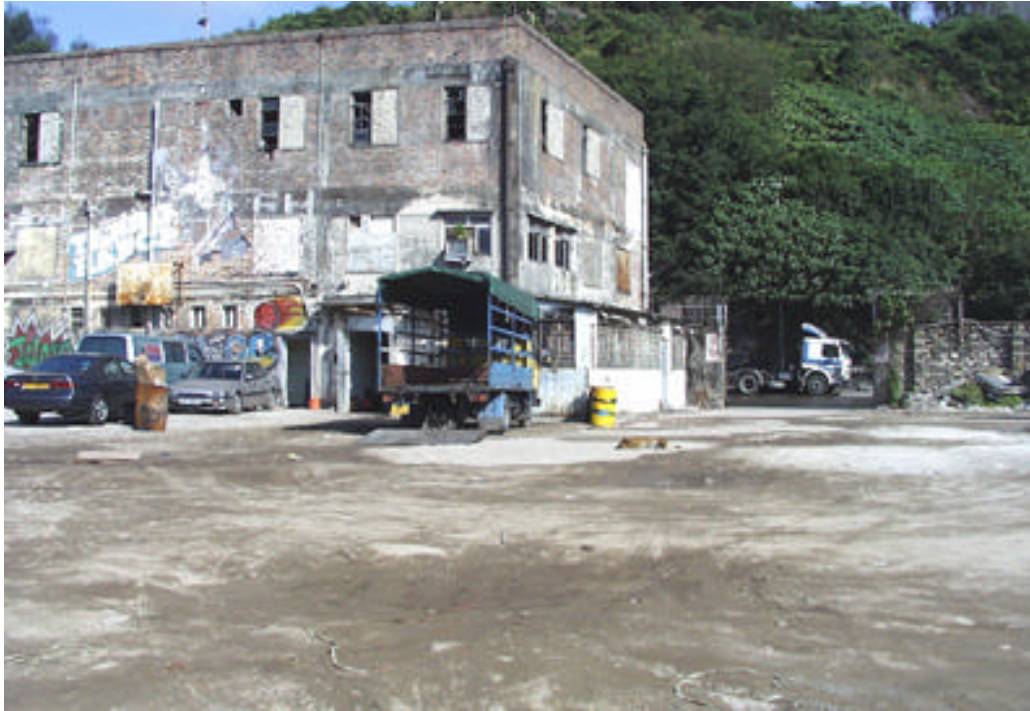
Photo 56 YTML 32-33 : The only entrance for the lot (5 Dec 98)
