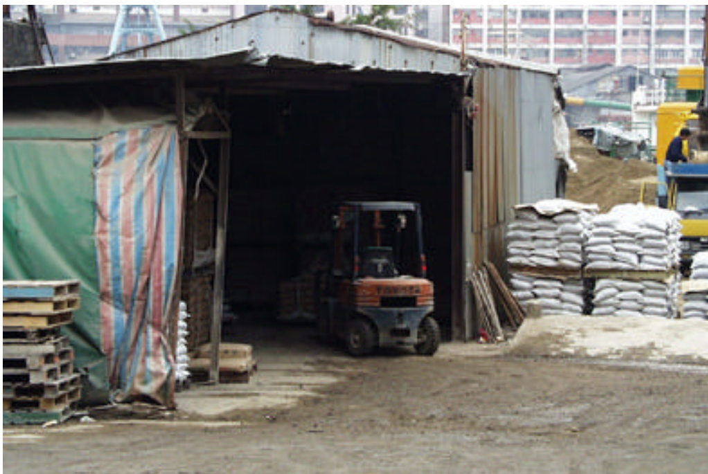
Photo 63 YTML 34 : Operating building material storage (24 Dec 98)
