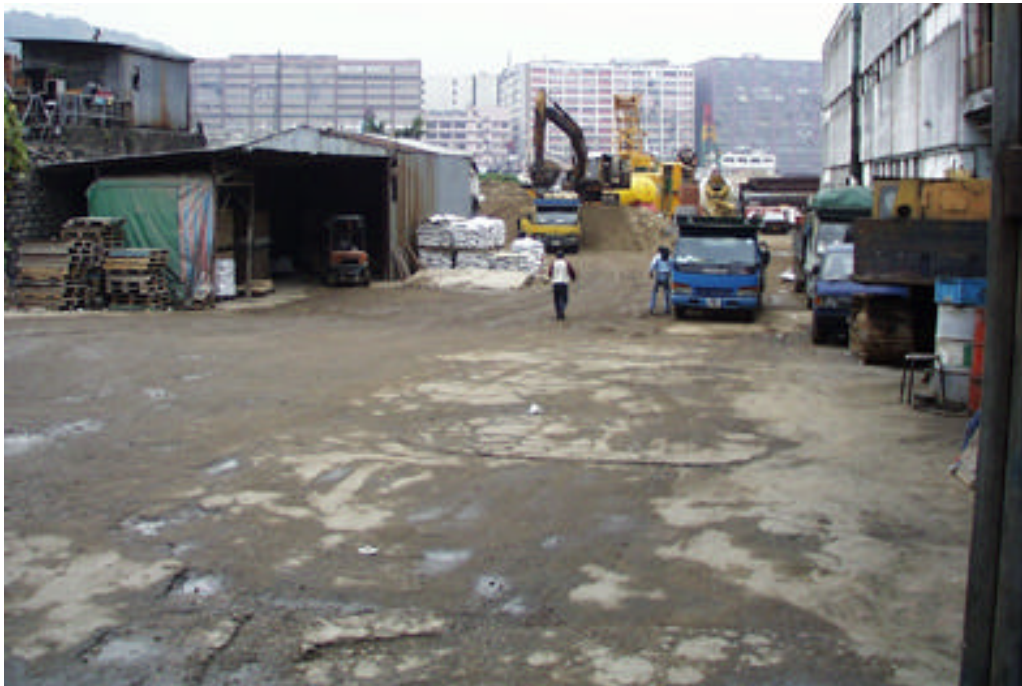
Photo 62 YTML 34 : Operating building material storage (24 Dec 98)
