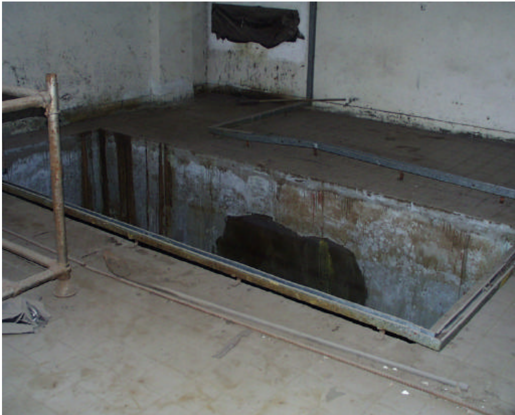
Photo 68 YTML 35 : A subsurface service bay in the vacated workshop (26 Jan 99)
