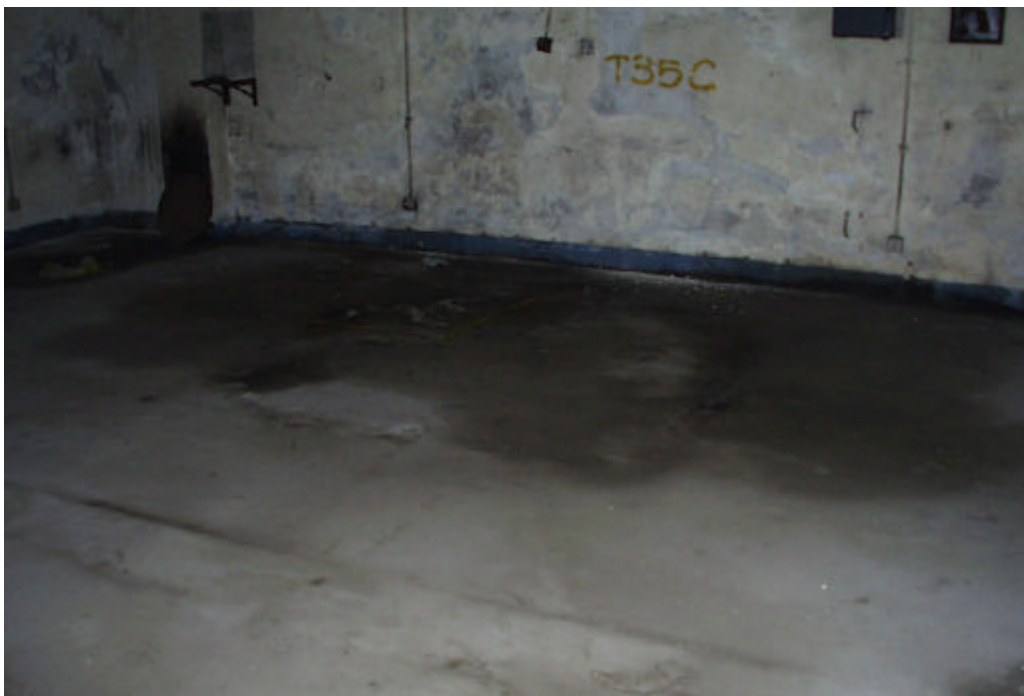
Photo 67 YTML 35 : Vacated machinery repair workshop (26 Jan 99)
