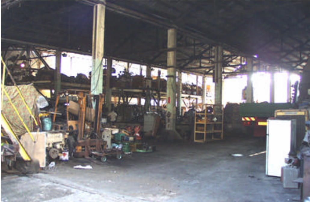
Photo 69 YTML 36-37 : Machinery repair workshop (5 Dec 98)
