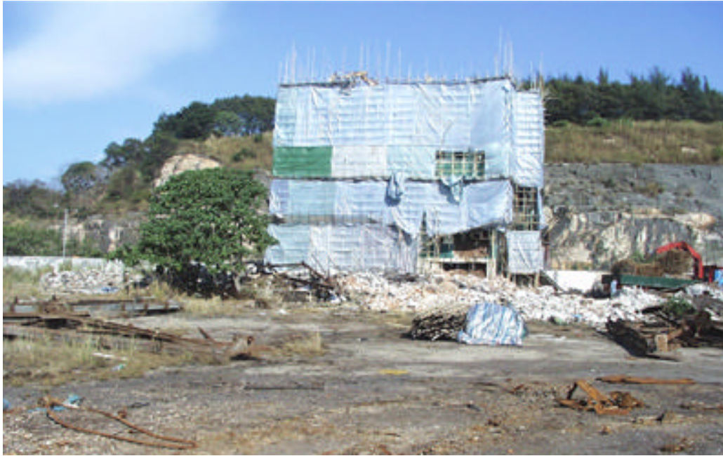
Photo 79 YTML 41-43 : Former ship repair workshop under demolishing (5 Dec 98)
