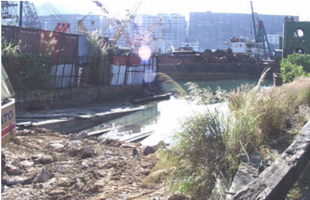
Photo 83 YTML 41-43 : Vacated jetty of the former ship repair workshop (5 Dec 98)
