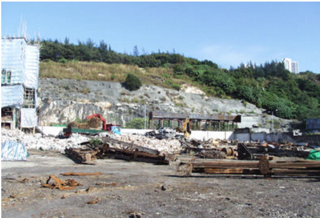
Photo 80 YTML 41-43 : Former ship repair workshop under demolishing (5 Dec 98)
