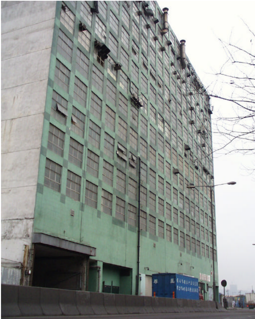
Photo 95 YTML 73-74 : Existing Industrial Building at Site (17 Mar 99)
