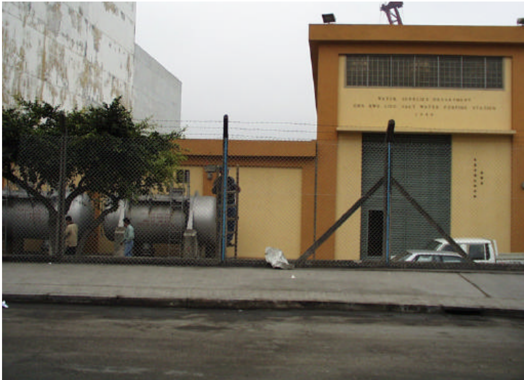
Photo 98 Existing Salt Water Pumping Station (17 Mar 99)
