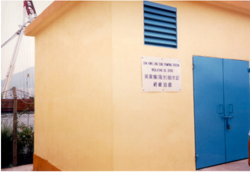
Photo 100 Insulated Oil Store Outside the Pumping Store (17 Mar 99)
