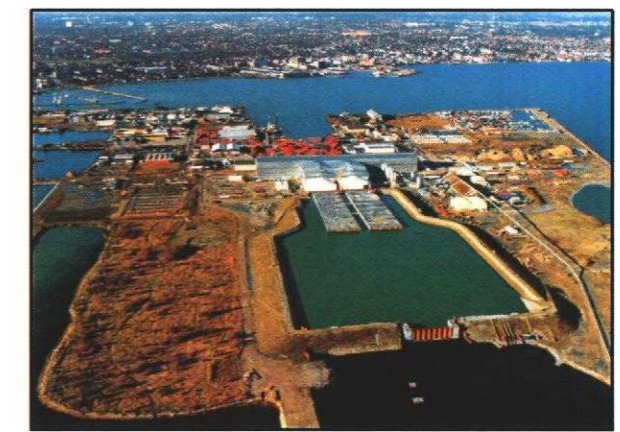
(CASTING BASIN FOR IMMERSSED TUBE TUNNEL OF ØRESUND FIXED LINK) - LARGE AREA FOR CASTING BASIN AND STORAGE OF PRECAST UNITS ARE REQUIRED FOR IMMERSSED TUBE TUNNEL OPTION.
