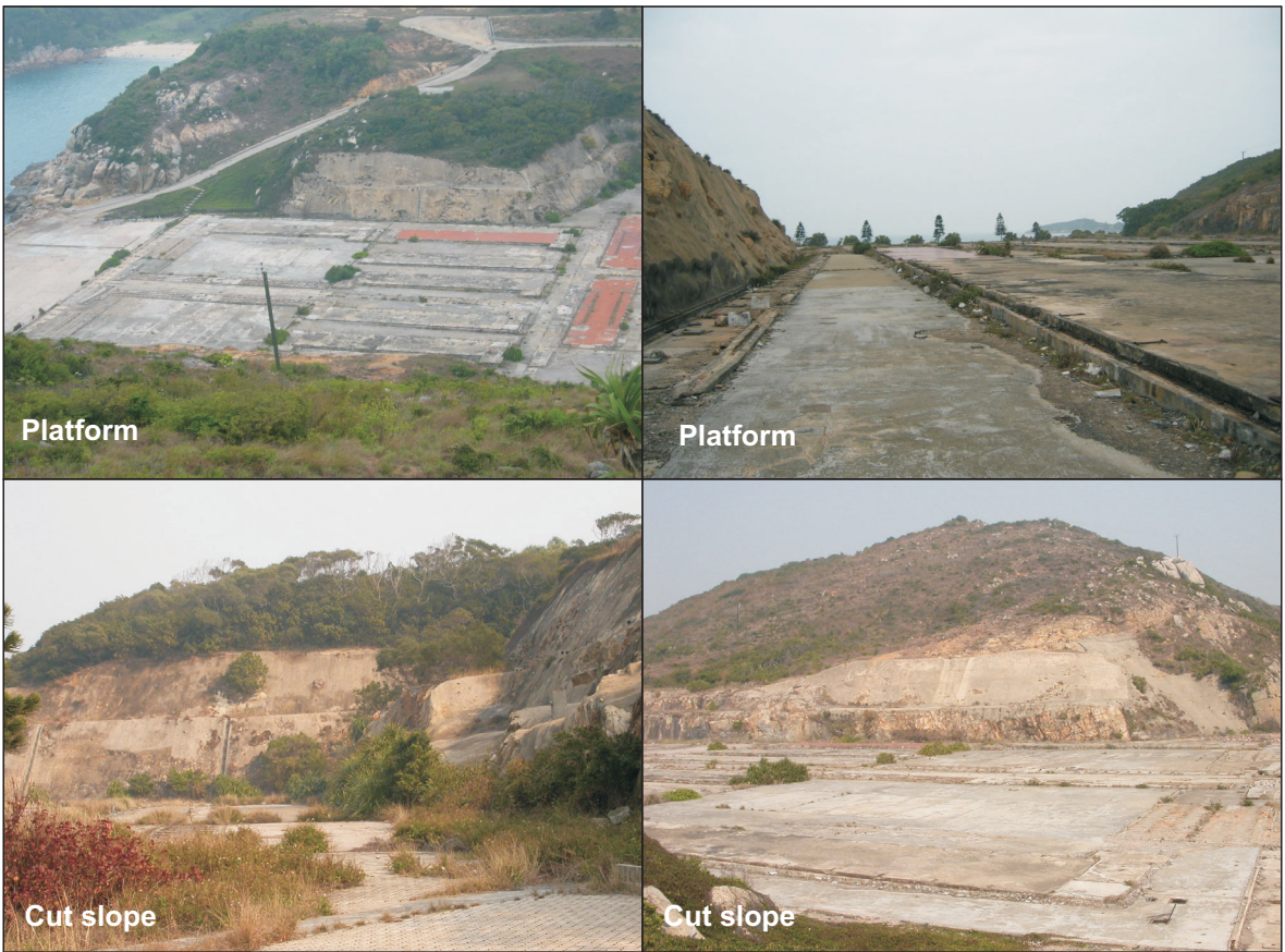
Figure 1.6 Existing Condition of South Soko (Photographs Taken in 2004)
