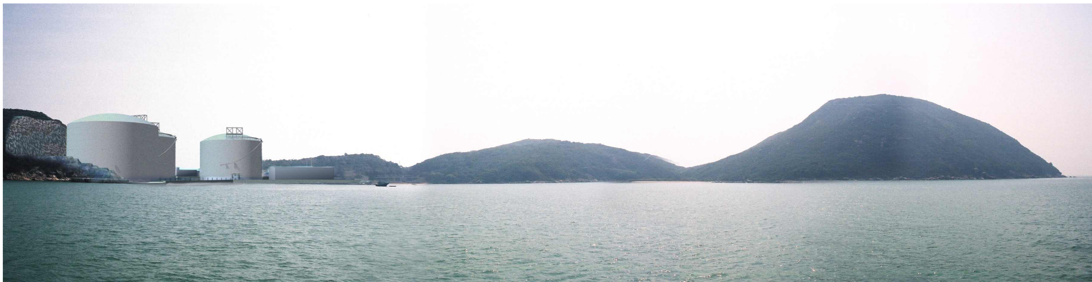
VIEW DISPLAYING THE 3D MODEL OF THE PROPOSED DEVELOPMENT DAY 1 Without MITIGATION MEASURES
