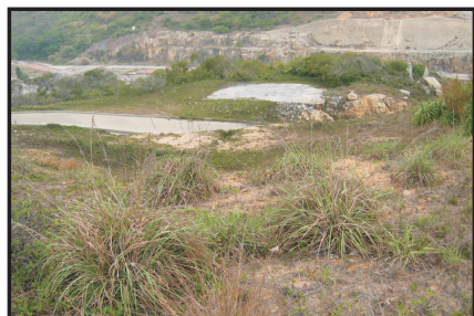
Concrete paths leading to the helipad were found within the grassland.
