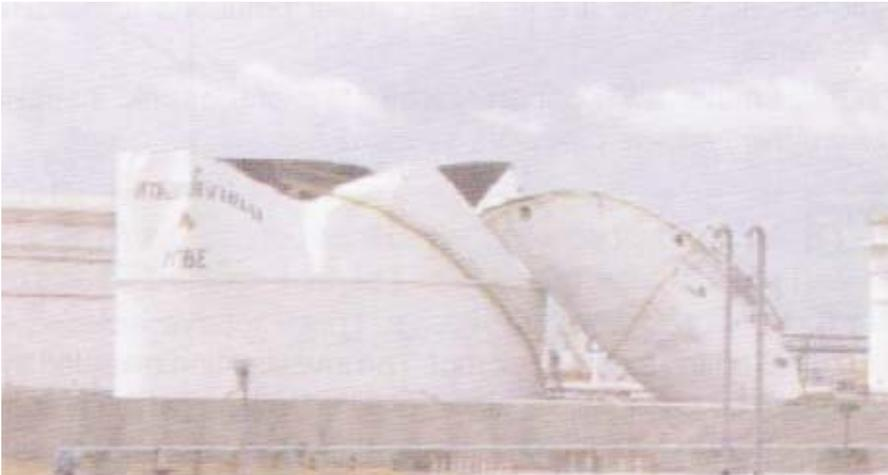
**Figure 4** - Example of rupture of a poorly-maintained tank
