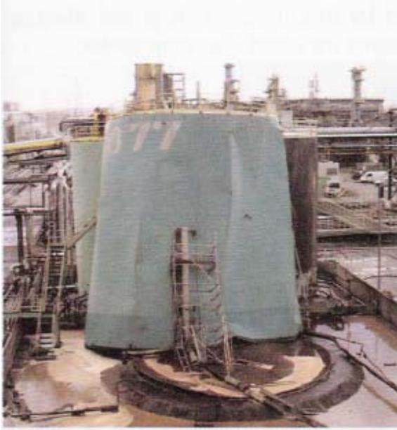
**Figure 3** - Tank internal explosion caused by lightning strike (BP, 2005b)
