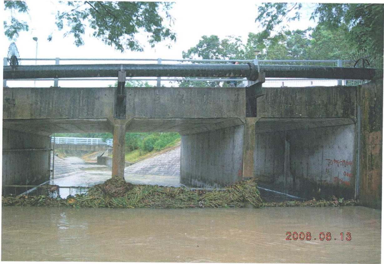
Photograph taken from Viewing Point B
